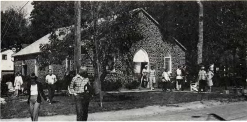
Short sections of cedar rail, set edgewise in mortar, give the chapel its unique appearance, both inside and out.
