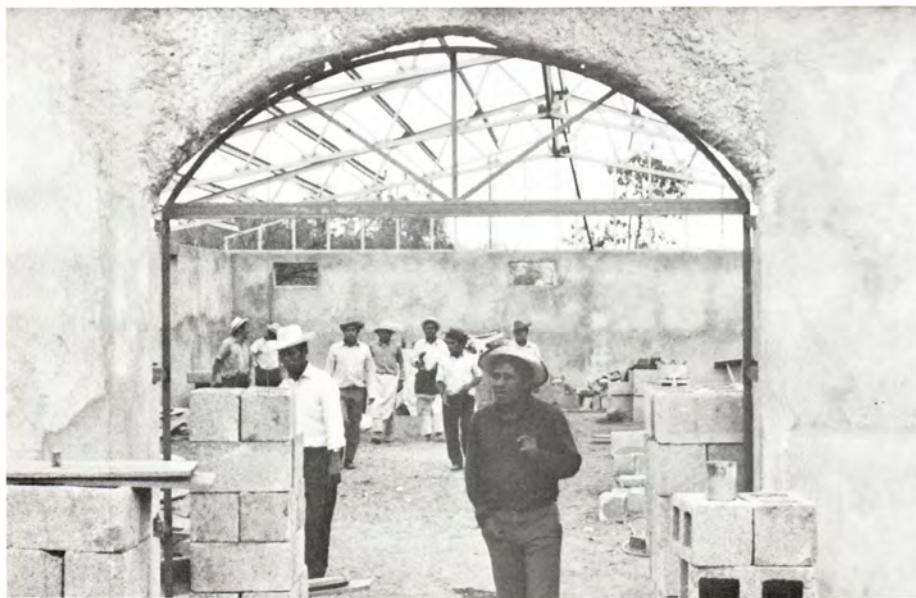
Steel roof trusses going in at Comalapa.
