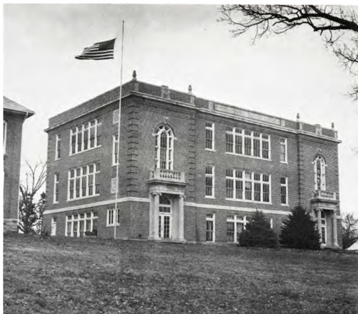
The three-story classroom/hospital building, with the administration building at the left.
