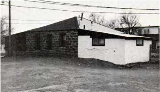
LEFT: The old stone house, with the adobe house beyond it.
