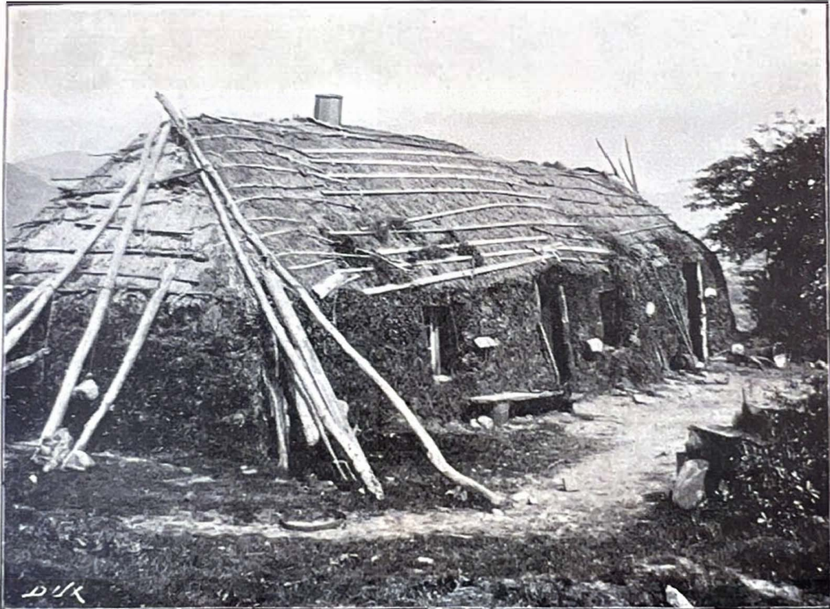
From a Photograph. A CROFTER'S COTTAGE IN THE NORTH OF SCOTLAND.
