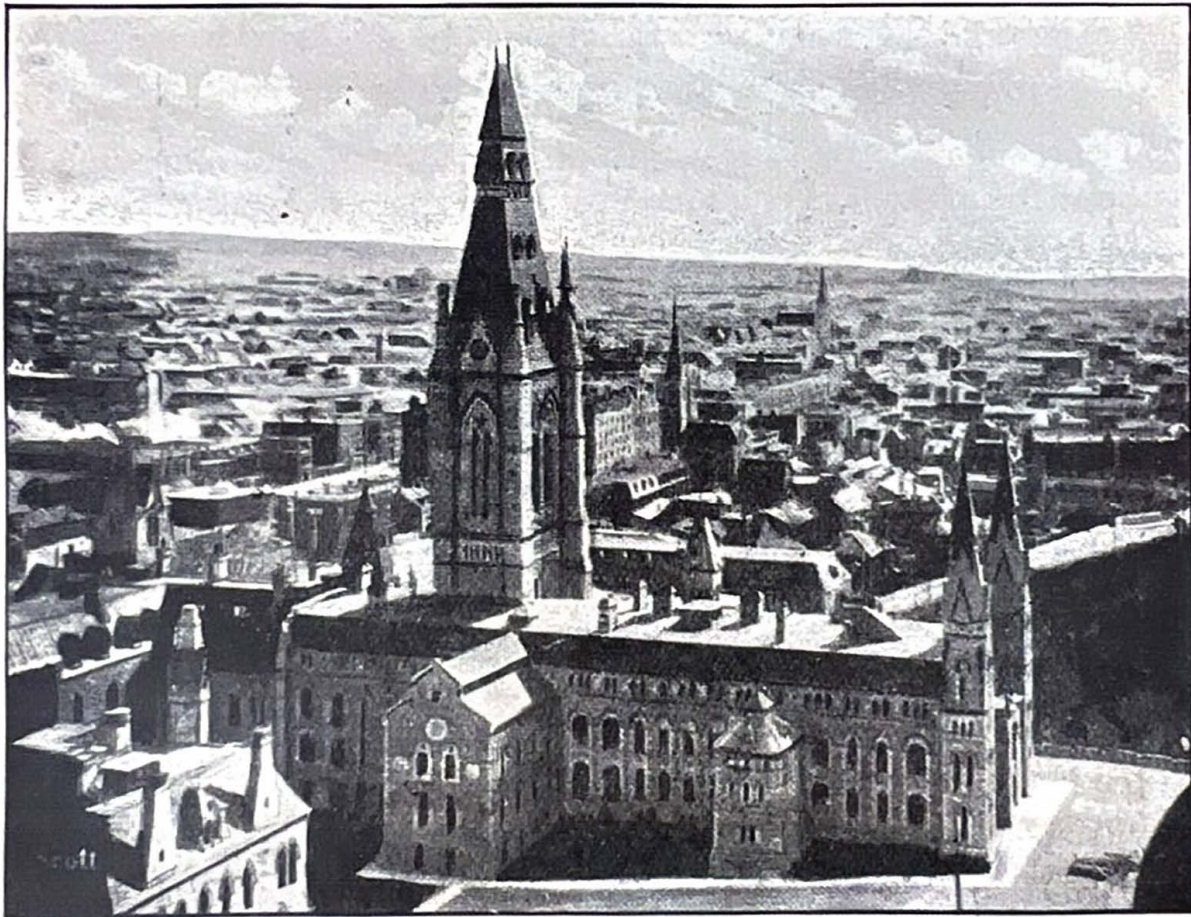
VIEW OF THE WESTERN SECTION OF OTTAWA CITY, CANADA.
